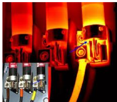
Fig. 2 IR vs. visual inspection, highlighting the importance of IR real thermal management
